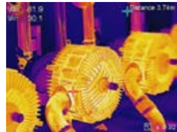
Mechanical Equipment Inspections
